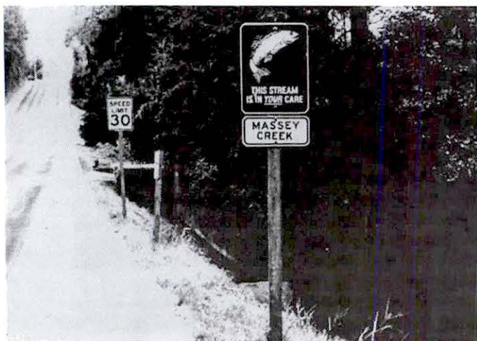
culvert carries Massey Creek crosses underneath 20th Ave. S.
